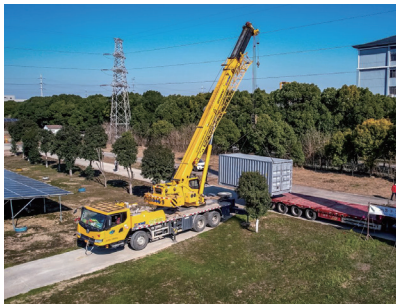
② Hoisting in Position
